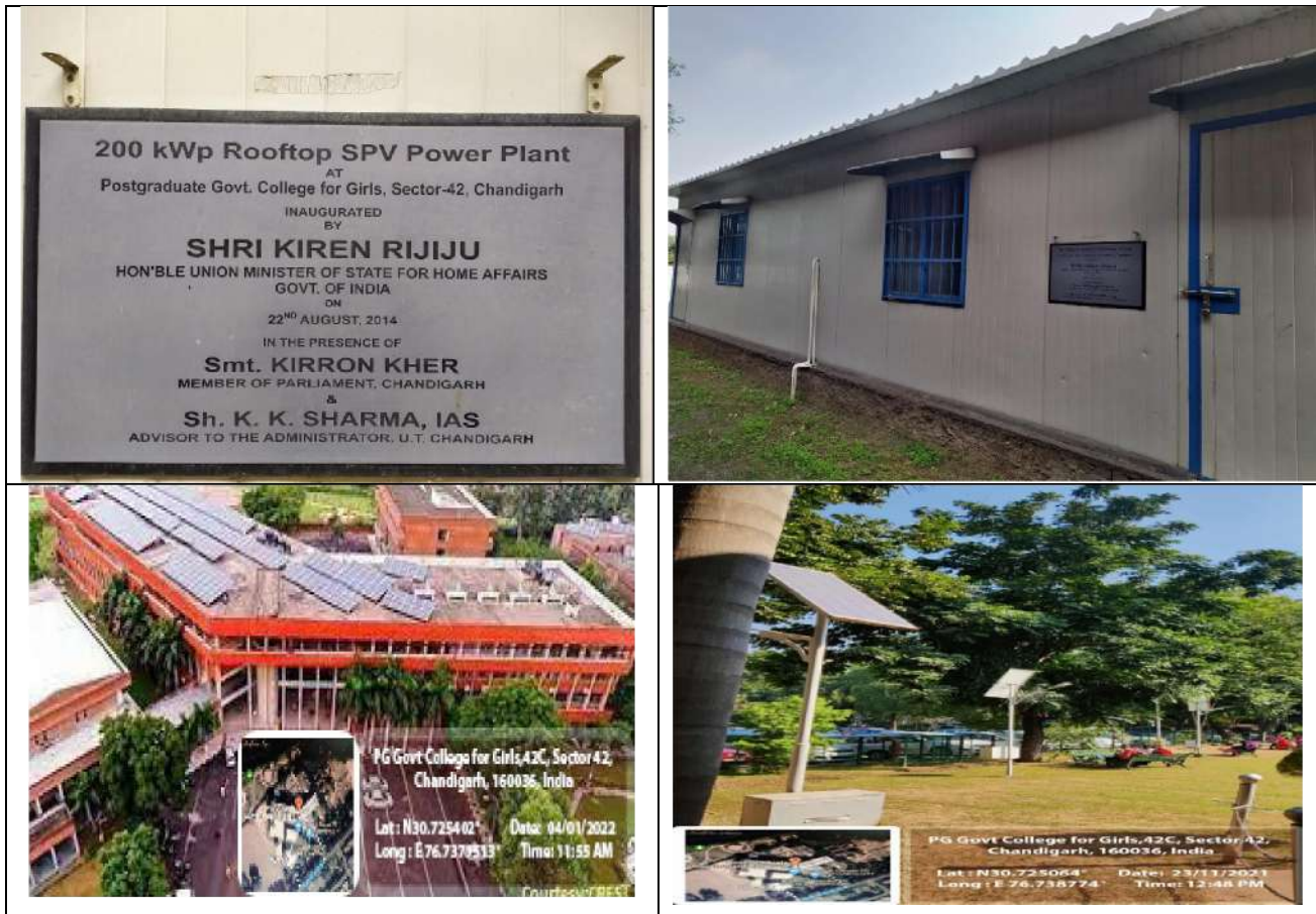
Fig 18: Solar Power in College Campus
