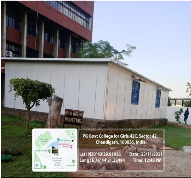
Rain Water Harvesting Units
